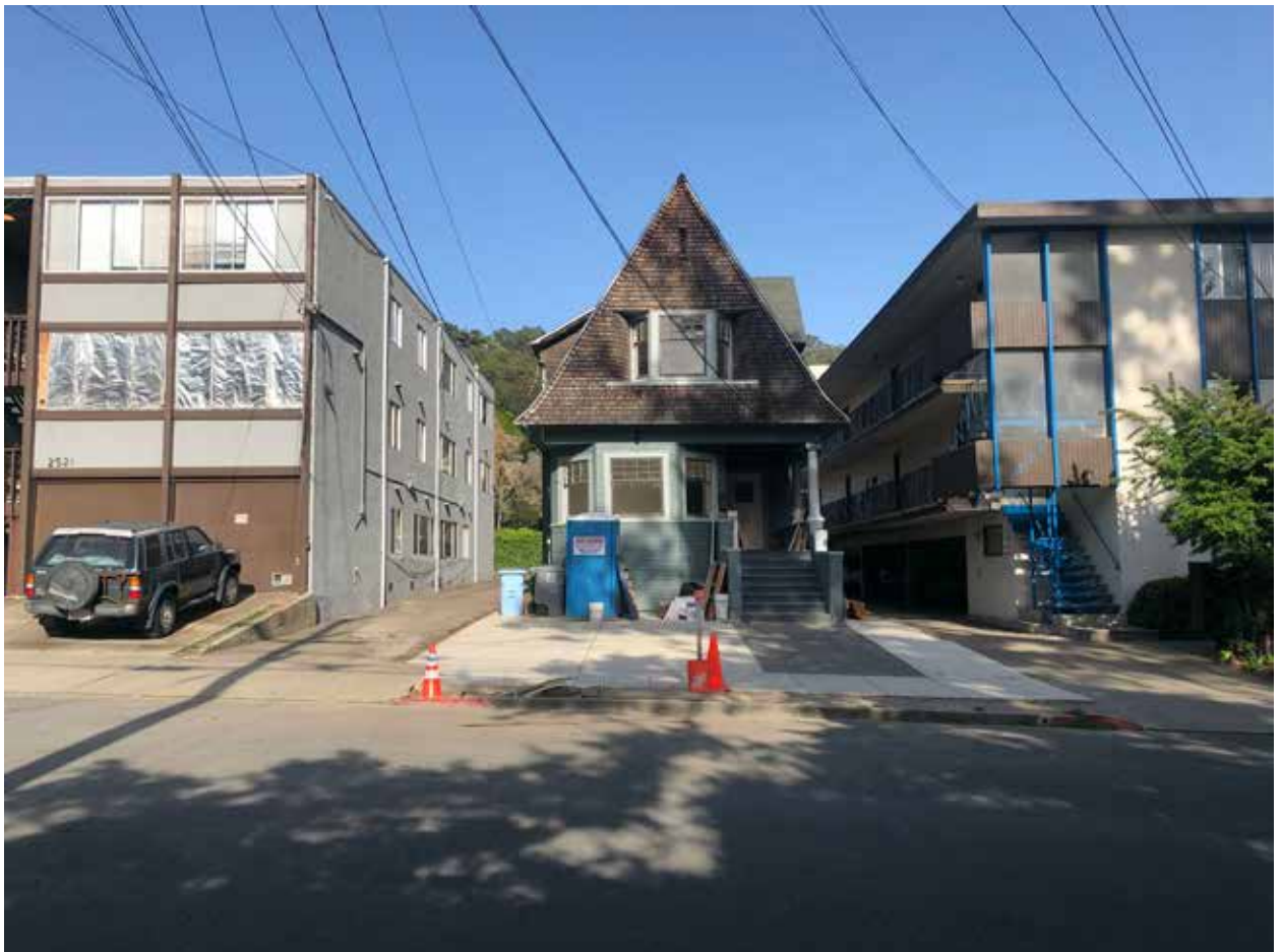
Fig.2 – 2523 Piedmont Ave. – Front (west) from avenue (figs.2-11, MH 2022)
