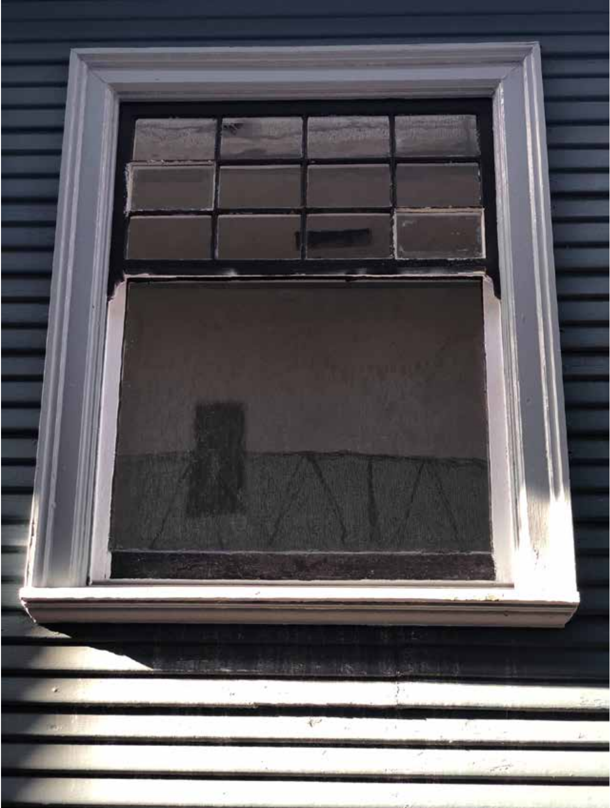
Fig.11 – 2523 Piedmont Ave. – Existing and typical wood window, casing, horizontal board siding
