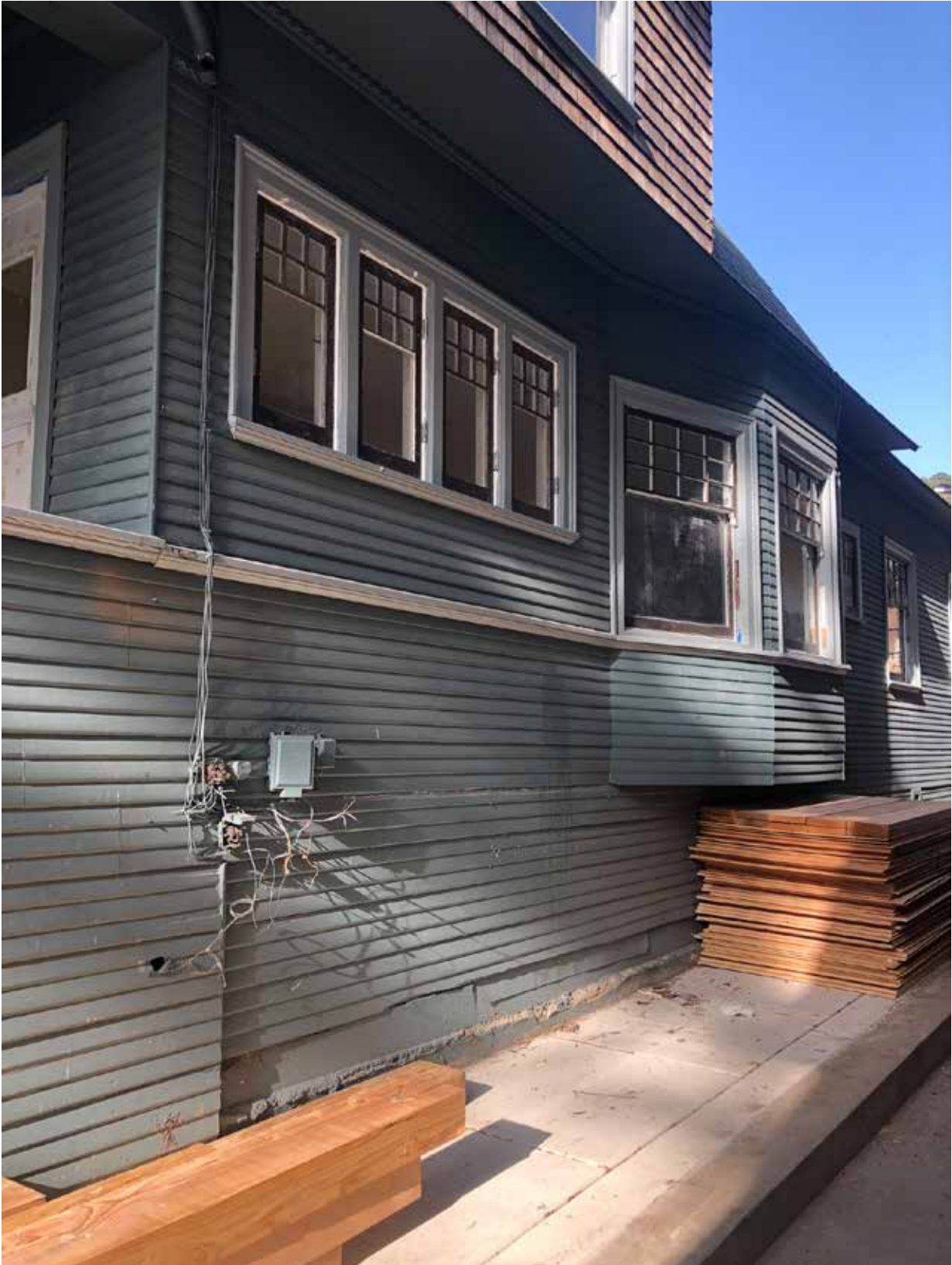
Fig.6 – 2523 Piedmont Ave. – Existing south side
