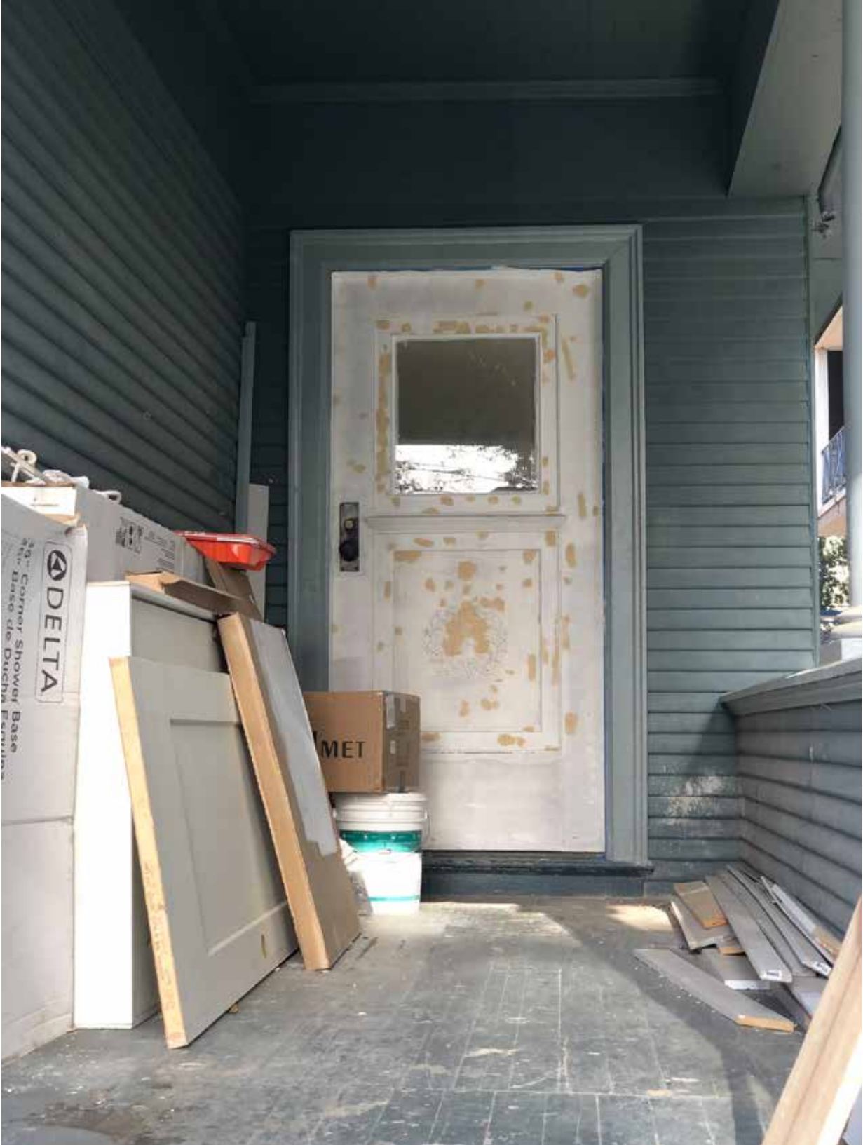
Fig.10 – 2523 Piedmont Ave. – Existing front entry door
