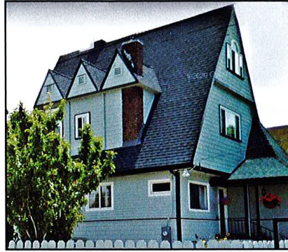
Fig.19. The earliest known true High-Peaked Colonial Revival house, at 2354 East 23rd Street in Oakland, designed by Hugo Storch in 1895. Google Street View.
