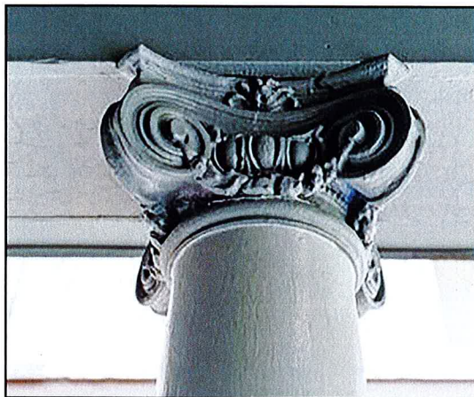
Fig. 8. An Ionic capital on a porch column. The Grubb Company listing photo, 2021
