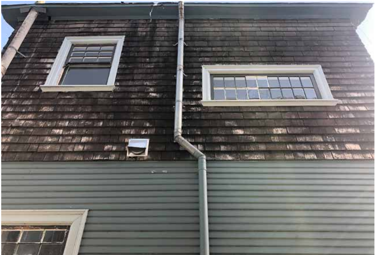
Fig.9 – 2523 Piedmont Ave. – Existing upper gable at north side
