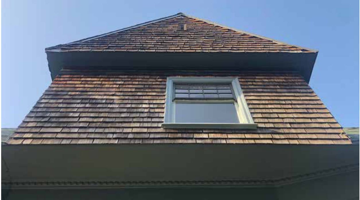
Fig.8 – 2523 Piedmont Ave. – Existing upper gable at south side
