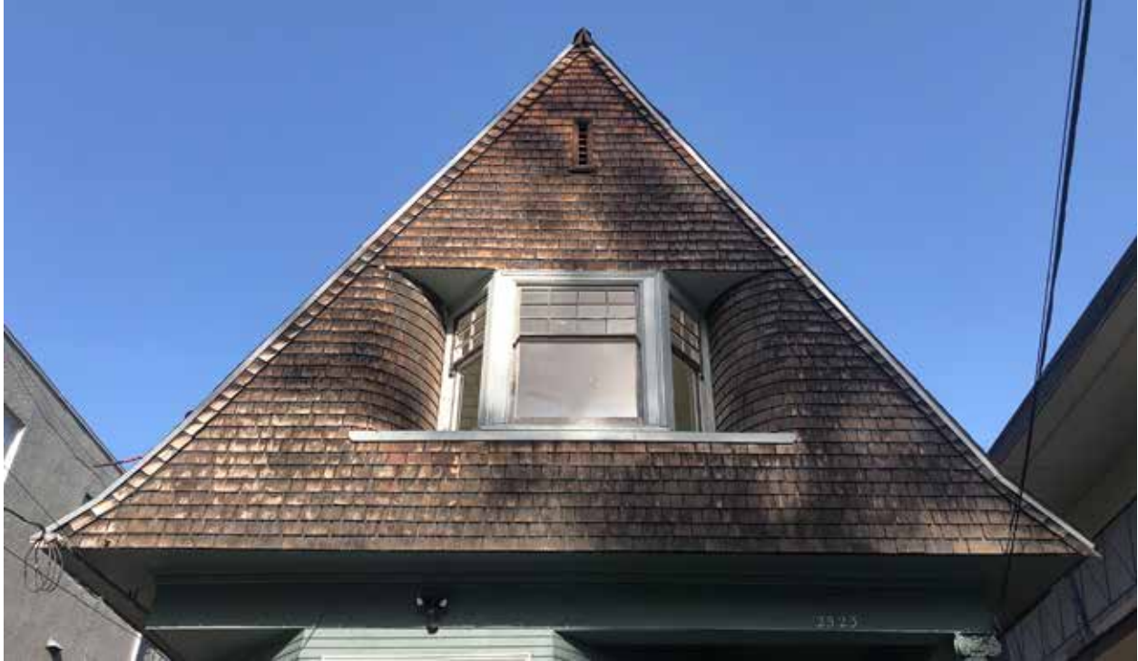
Fig.3 – 2523 Piedmont Ave. – Existing upper front (figs.1-9, MH 2022)
