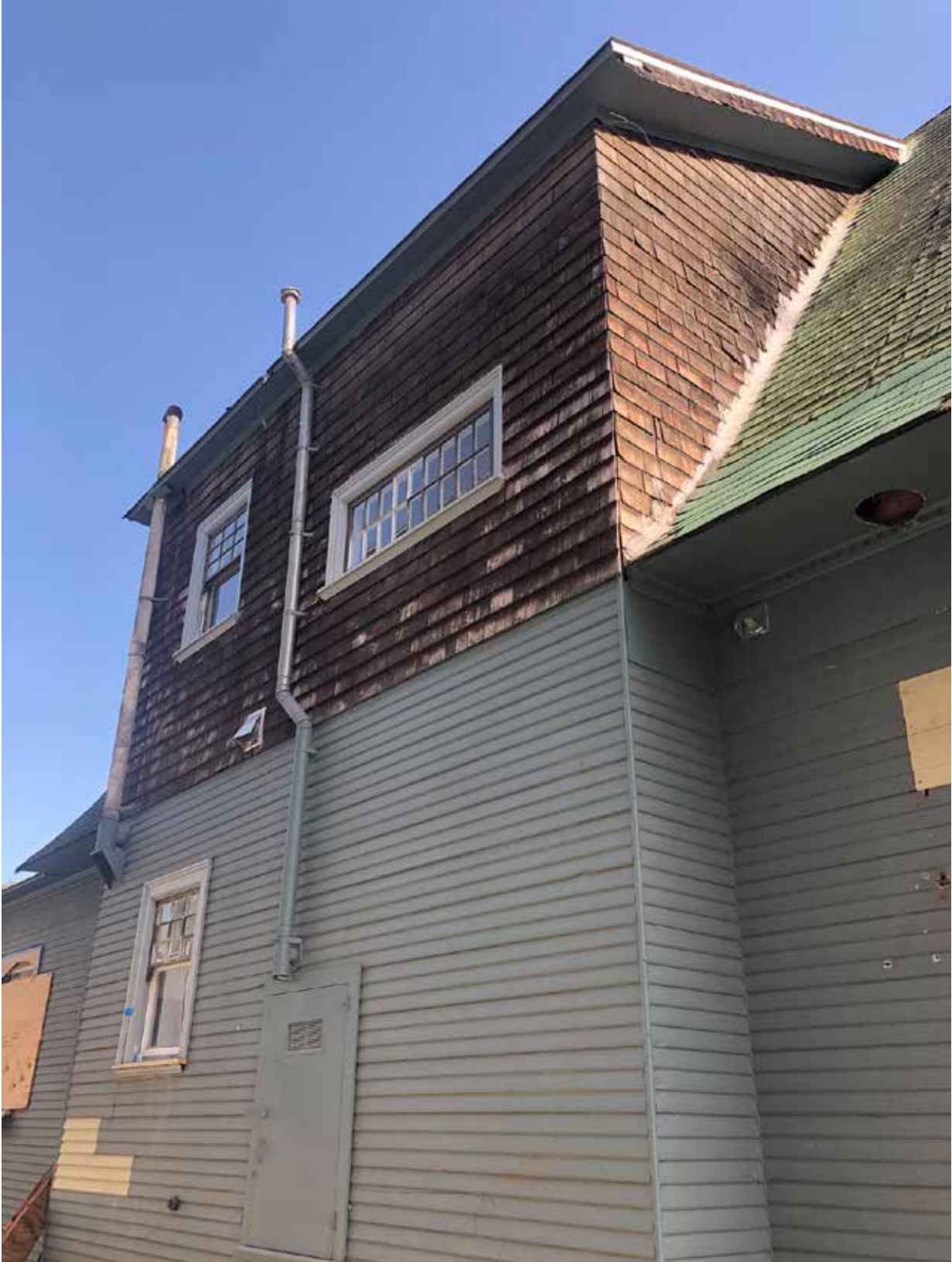
Fig.7 – 2523 Piedmont Ave. – Existing north side (part)
